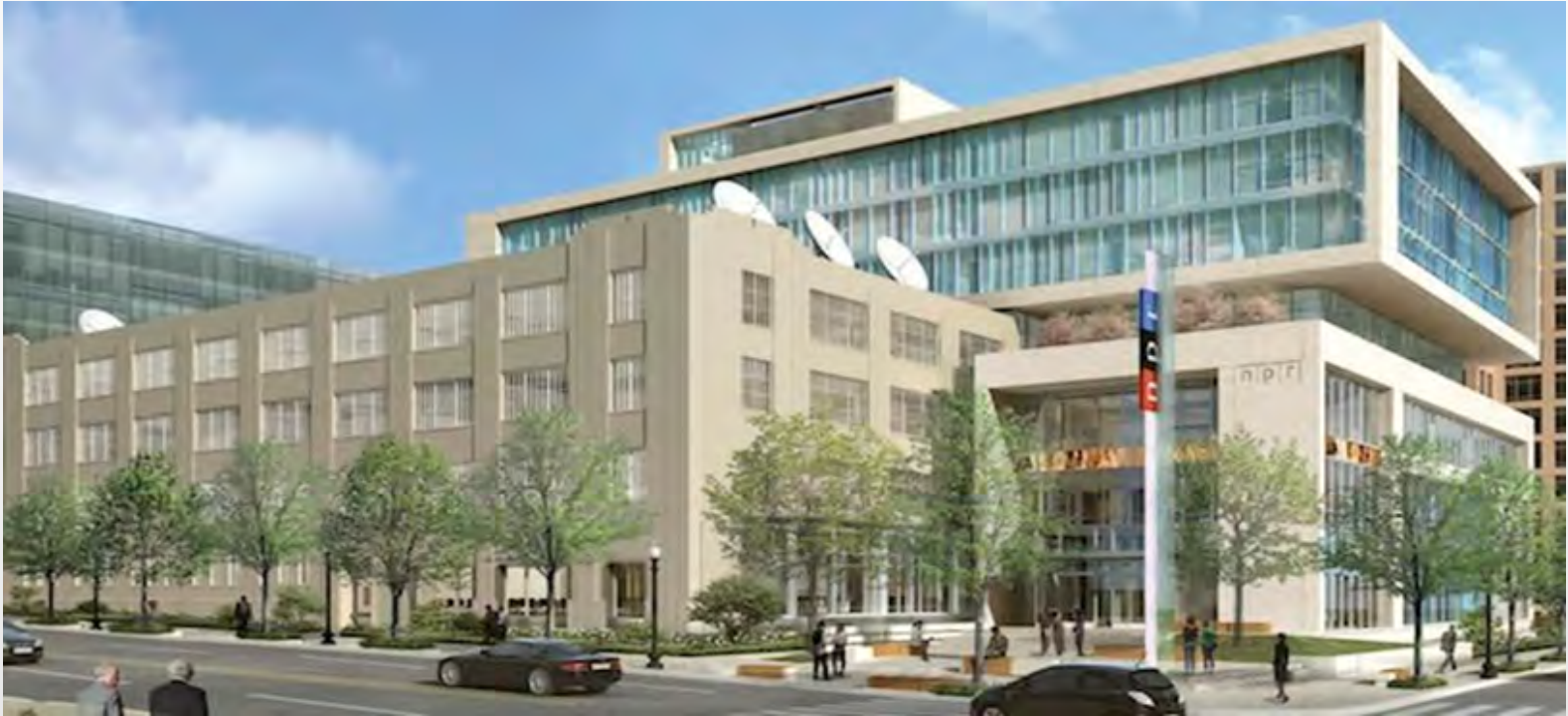
Building Mounted Dish Antennas
