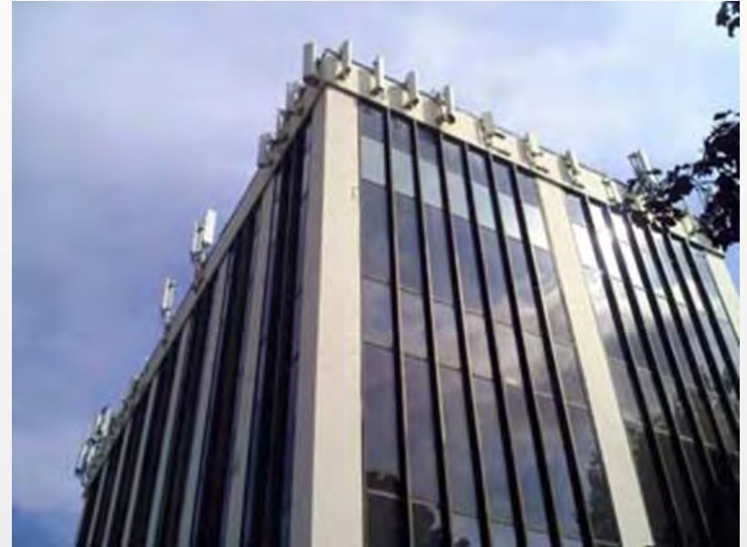
Building Mounted Panel Antennas
